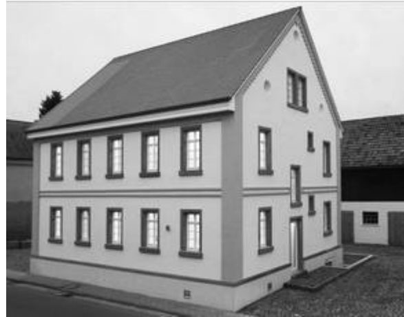
Photo 26: After modernisation: A Passive House
